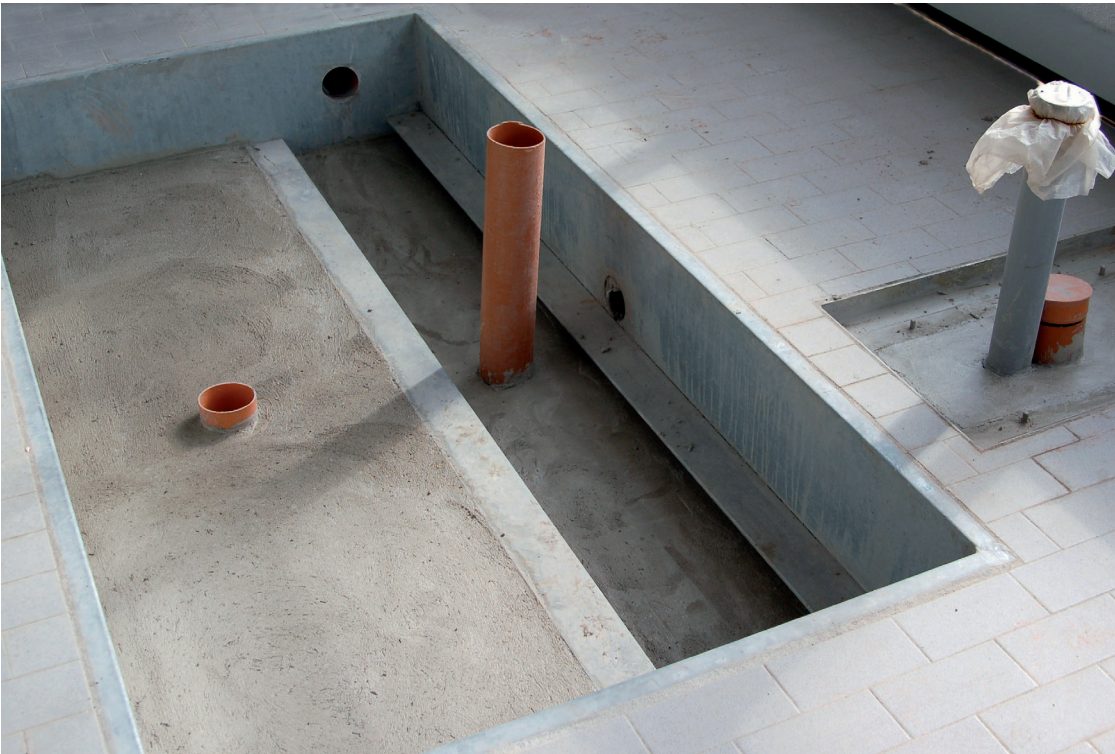
Fig. 31: Assembling case concret-casted (example)
